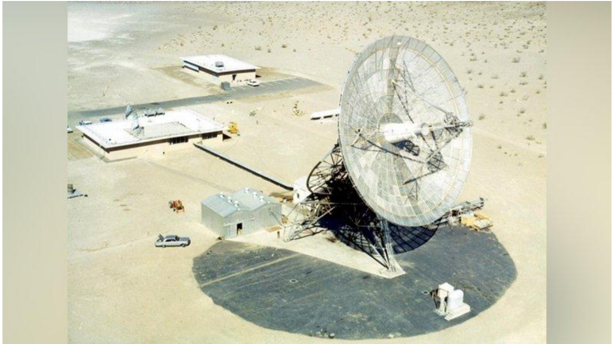
The Pioneer Station (DSS-11), a 26-meter polar-mounted antenna was the first deep space antenna to be constructed at Goldstone. Completed in 1958 in time to support the Pioneer 3 mission, DSS-11 became the prototype antenna for the Deep Space Network. Image Credit: NASA/JPL-Caltech
